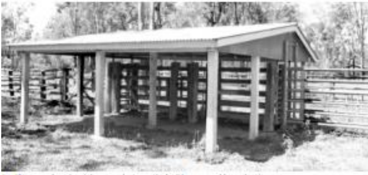
Figure 3. Handling Facilities Covered with roof
